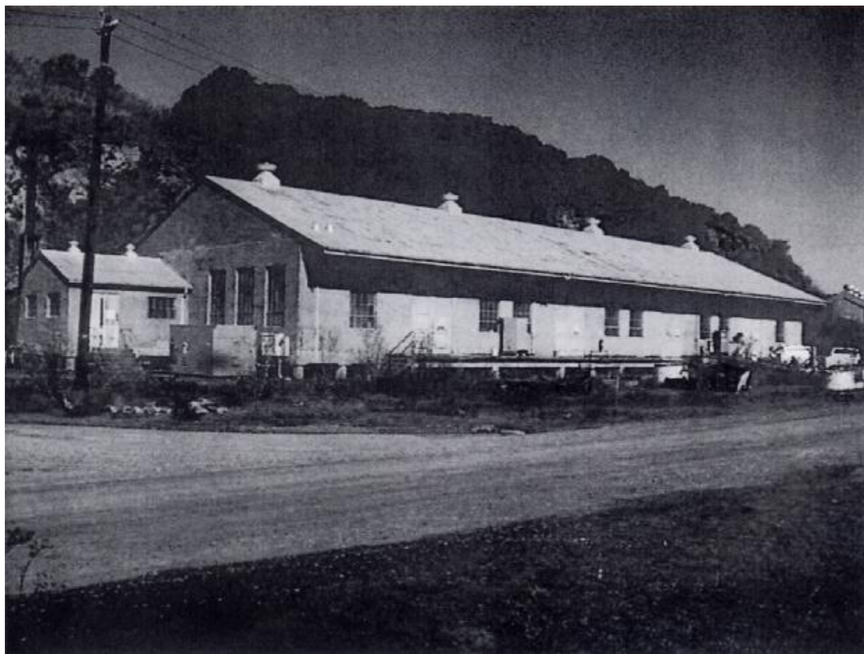
Figure 7. Building A259 at Mare Island, Ca.
